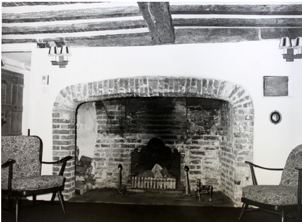
One of the brick fireplaces with its four-centred arch construction. The photograph was taken in 1978.
